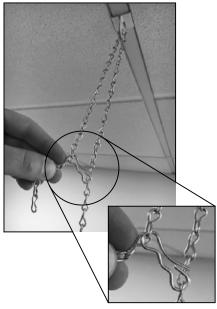
STEP 5: Repeat STEPS 3-4 for installation of chain on right side.
